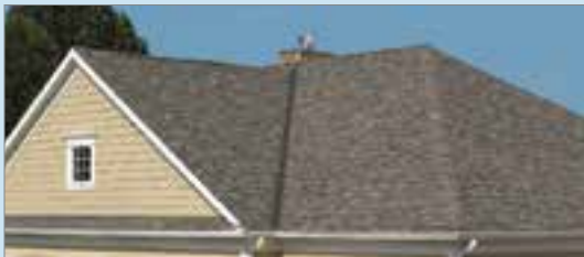
Roofing and Ventilation
