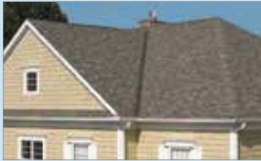
Roofing and Ventilation
